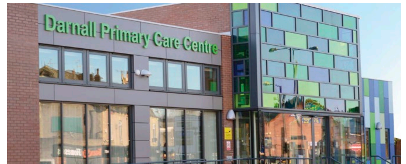
New Darnall GP practice building
